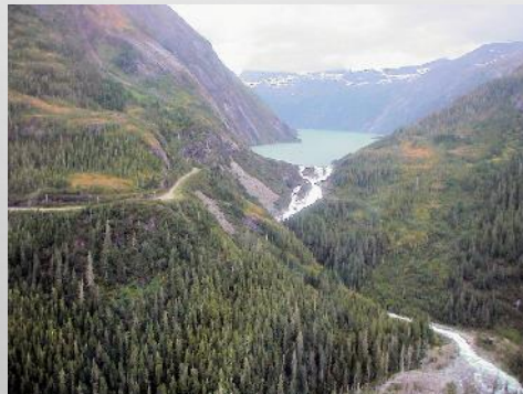
Long Lake, lake tapped (Snettisham Hydroelectric near Juneau)
